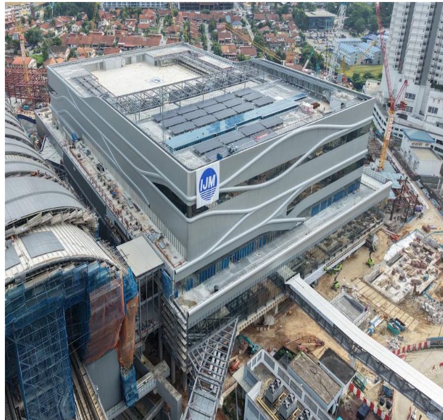
Johor Bahru–Singapore RTS Link ICQC complex
